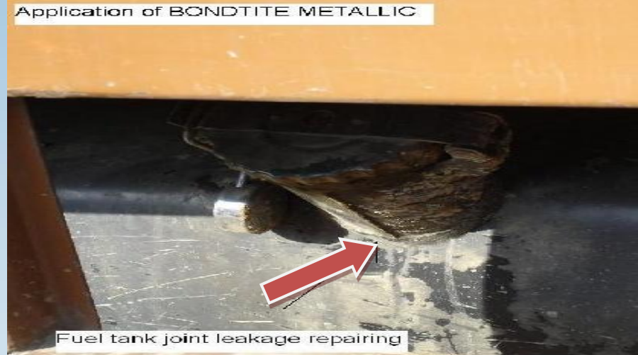
Fuel tank leakage repairing
